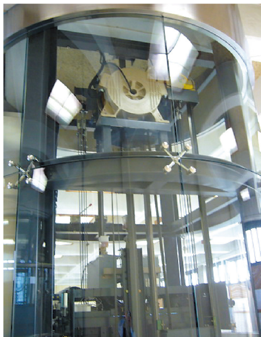
桃園國際機場第一航廈觀光梯，永磁同步無機房主機 Permanent magnet synchronous roomless winch of Taiwan Taoyuan International Airport terminal 1 tourist elevator.
