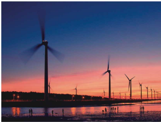
2000hp永磁同步風力發電機，內部構造直徑3公尺，釹鐵硼磁鐵8500片(2000kg) 1.5MW wind power permanent magnet synchronous generator, its internal diameter is 3 meters, NdFeB magnet containing a total of 8500 pieces ( 2000kg ) .
